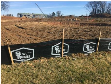
Ensure silt fence is dug into ground to prevent runoff from escaping underneath.
