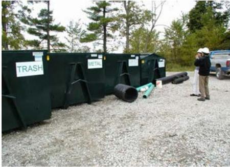
Waste management area is clearly designated away from construction activity. Use of separate containers (with lids) for trash, recycled products, etc.
