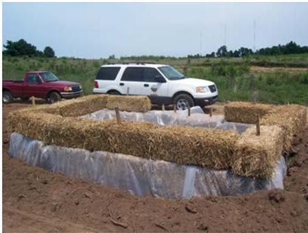
Concrete washout for single lot use made of straw bales and plastic. Washout is located away from pavement, storm drains, and ditches to ensure that any overflow does not move toward surface waters.
