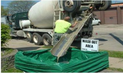
Washout area clearly designated with a sign, conveniently located for truck access, and plastic lining is free of holes and tears.
