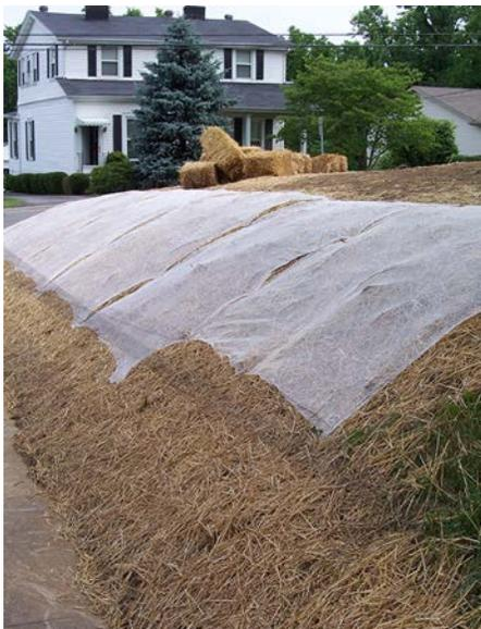
Slope stabilization using straw/hay mulch and mulch netting.
