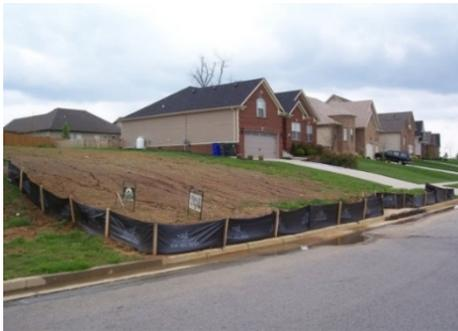
Site with properly installed silt fence. Note that fence posts are installed on the downhill side of the fabric.
