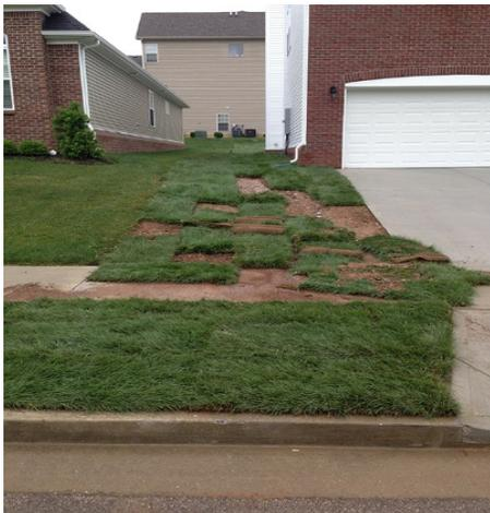
Sod installation failure. Sod needed staples. Photo credit: Barry Tonning, Tetra Tech
